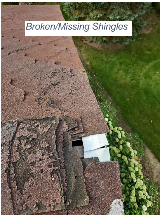
Visual verification of damage to roof at 8640 Gull Road
